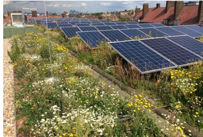
Green roofs increase solar panel efficiency
